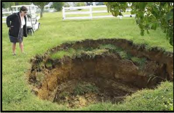
Sinkhole in Trinity, Alabama (Gary Lloyd)
